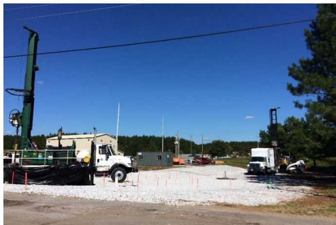
Figure 10. West Side Construction
