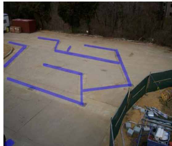
Figure 3. Electrodes and TMPs Installed Below Grade Allowing Unrestricted Access
