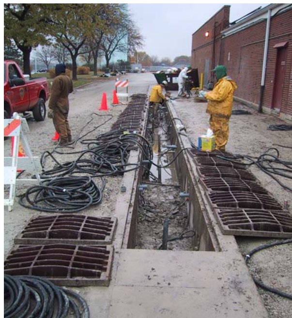
Figure 1. Installation of ERH Components in Common Utility Trench
