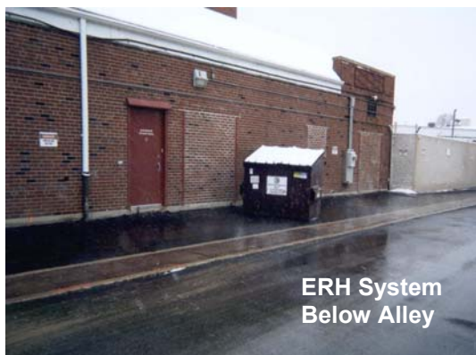
Figure 2. The Alley Remained Open during ERH Remediation
