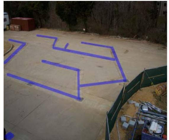
Figure 3. Electrodes and TMPs Installed Below Grade Allowing Unrestricted Access
