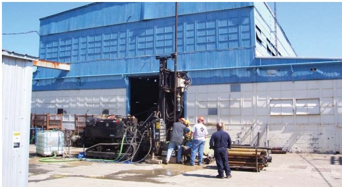
Figure 1. Mini Sonic Drilling Technique
