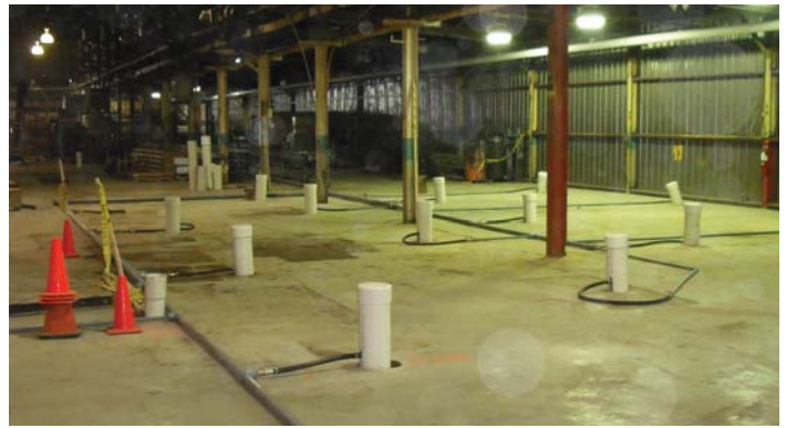
Figure 4. Completed NWD Area
