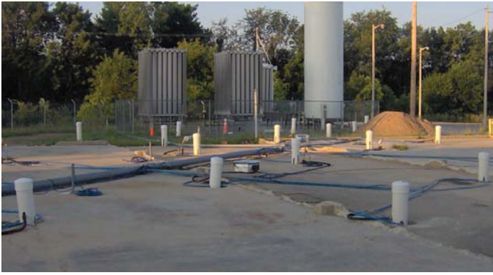
Figure 3. Completed UST Area
