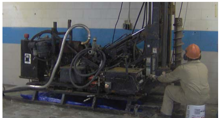
Figure 2. Limited Access drilling in the NED
