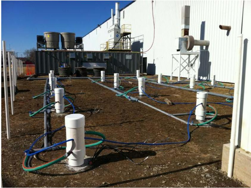
**Figure 3.** ERH electrodes and equipment compound
