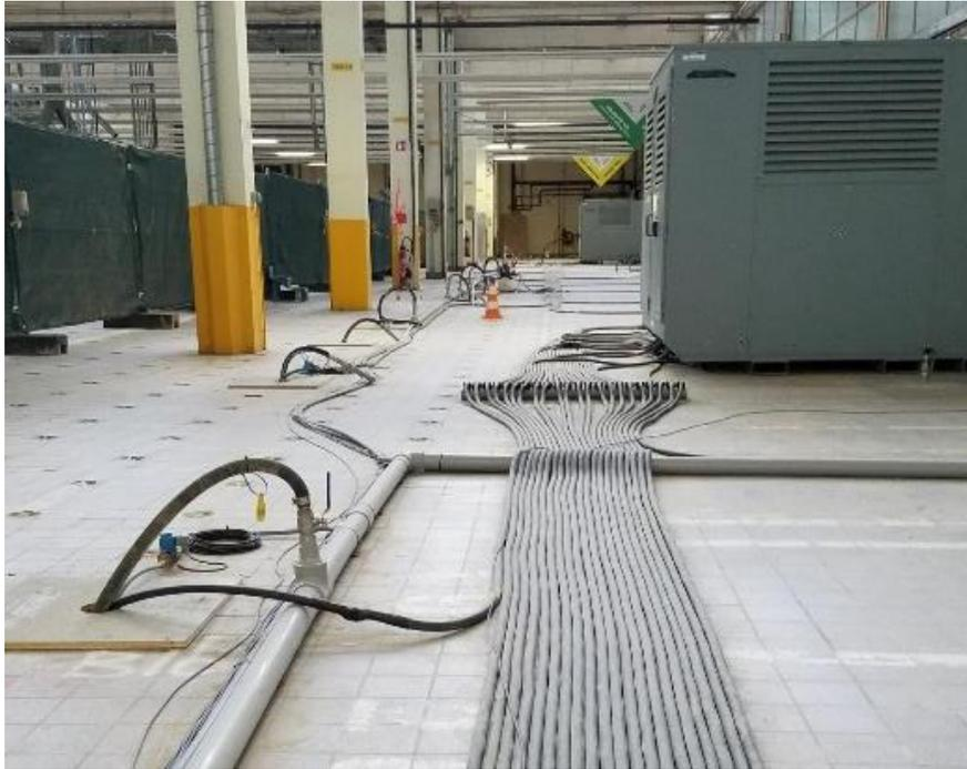
**Figure 2. Thermal remediation under an active manufacturing facility.**
