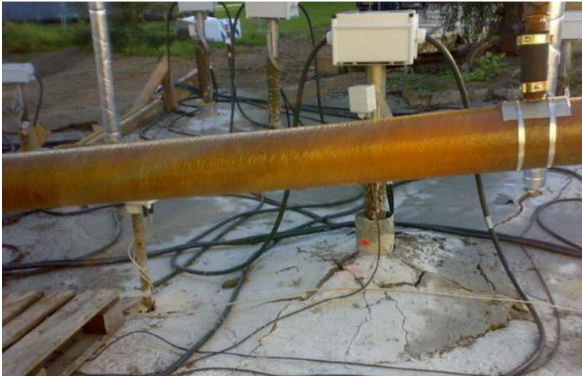
Figure 1. Subsidence observed at a PCE site with a thick peat layer heated to 100°C and dewatered (Skuldelev, Denmark; Nielsen et al. 2010).
