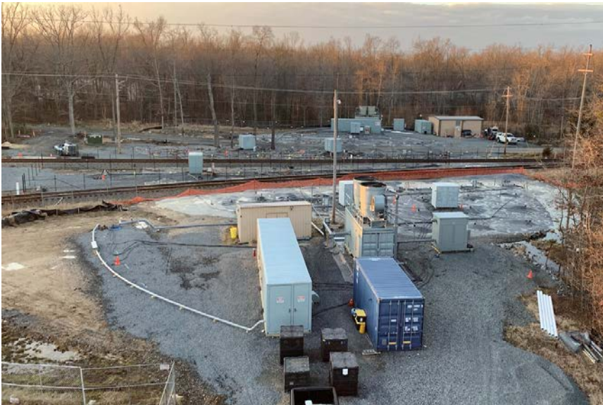
ERH electrode field construction
