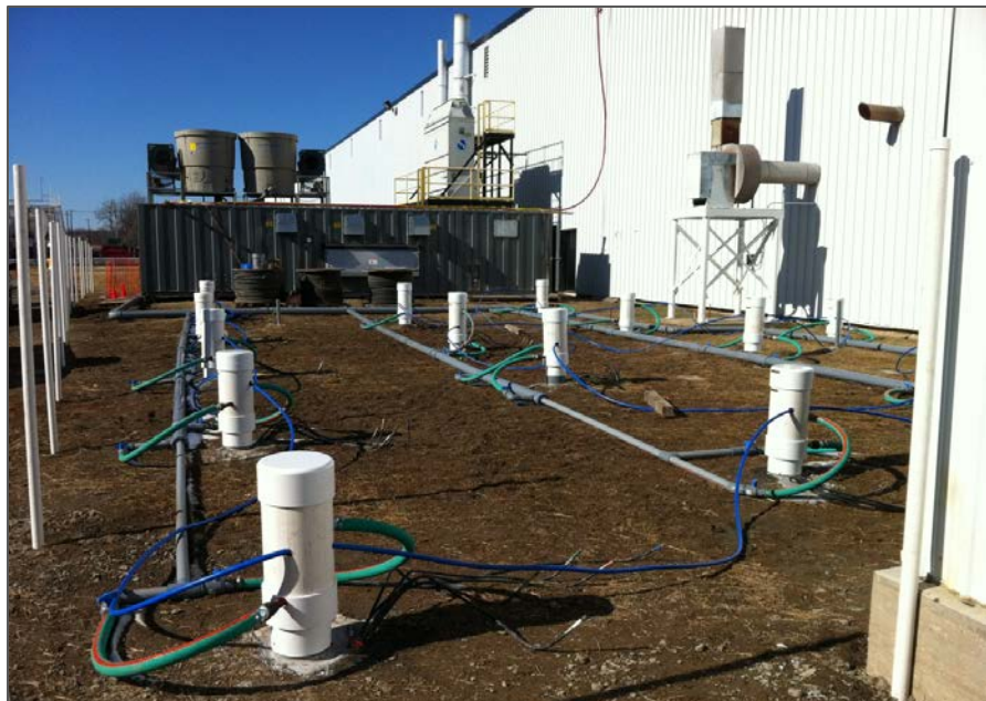
ERH electrode field construction
