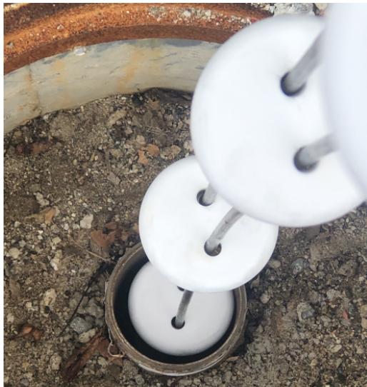
Figure 1. FlexHeater® element which provides flexibility to control power input
