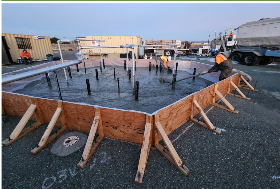
Installation of insulating concrete layer above treatment volume
