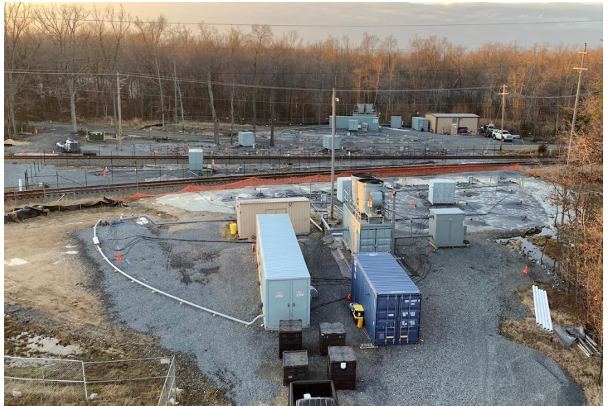
ERH Electrode Field Construction
