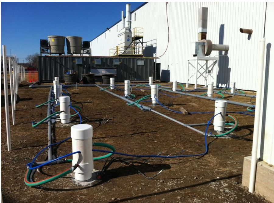
ERH Electrode Field Construction
