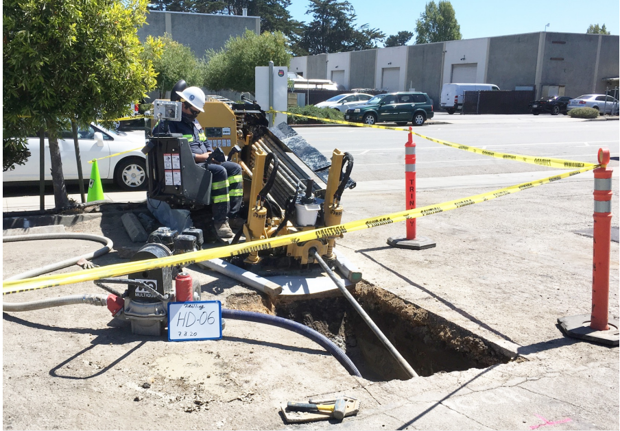
Horizontal Drilling
