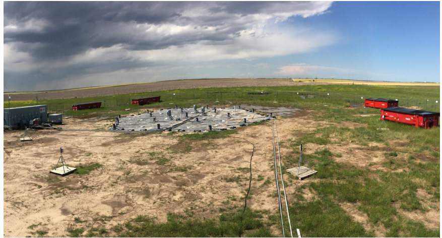
Panoramic Drone Shot of Site
