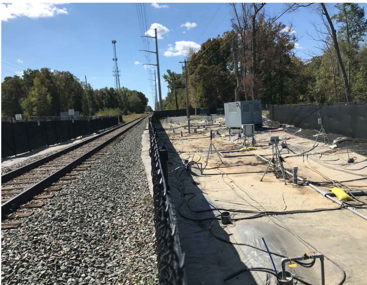
Figure 3: ERH operation under an active railroad- electrodes were placed under the railroad, and the subsurface was heated to boiling temperatures without any adverse impacts (Brandywine, MD; TRS Group, unpublished).
