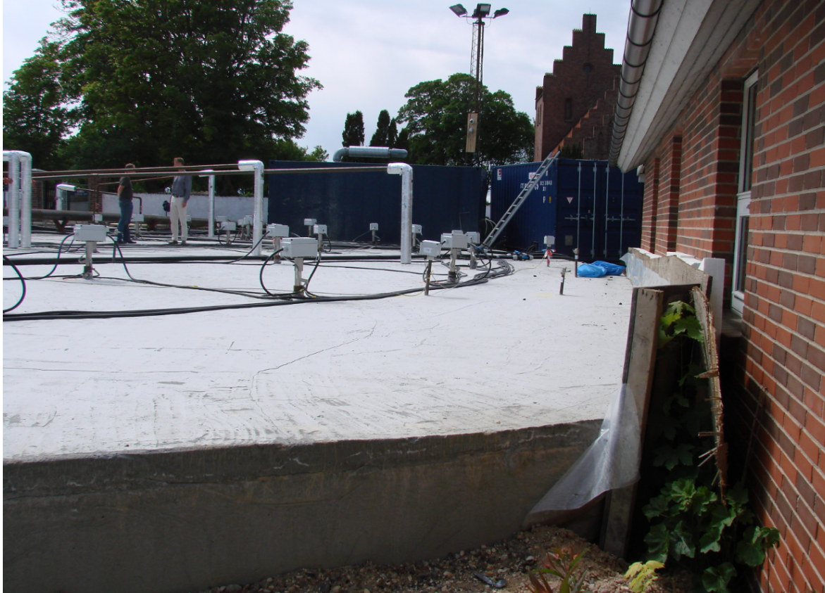
Figure 2: TCH remediation of a 9-meter-deep clay layer heated to 100°C next to a building-- no subsidence observed (Reerslev, Denmark; Kruger and TerraTherm, unpublished).
